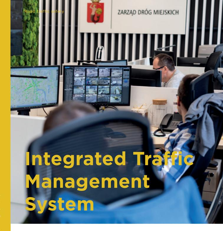
The Integrated Traffic Management System contributes to the improvement of traffic flow and safety. In Warsaw the system has been operating since 2008 and back then it covered 37 intersections. Today, it encompasses a total of 321 intersections. In 2018 another 53 intersections at Okopowa St., Żwirki i Wigury St., Puławska St., Wiertnicza St. and Powsińska St., among others have been added to the system.
